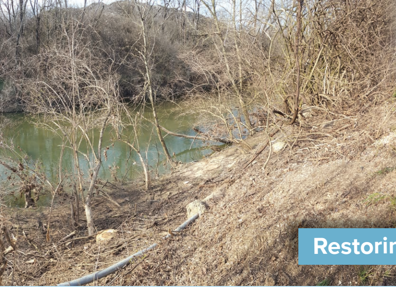
BEFORE - Steep unstable streambanks with dense shallow-root vegetation
