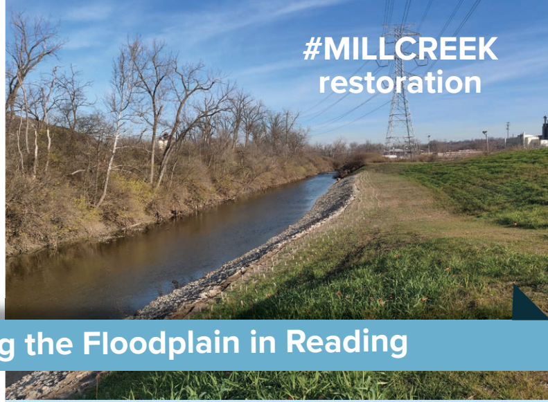
AFTER - Streambank stabilized, open and accessible to public, connected to the floodplain, and planted with hardy native plants
