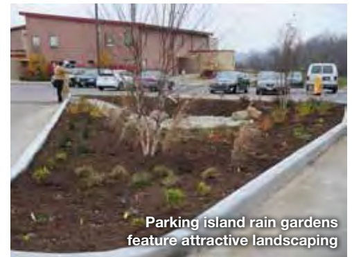
Parking lot runoff is filtered in the bioswales
