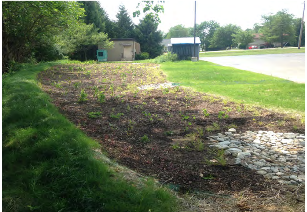
The bioswale pictured above filters stormwater runoff from the school's parking lot allowing pollutants, sediment, and nutrients to settle-out before the water enters the East Fork Mill Creek.
