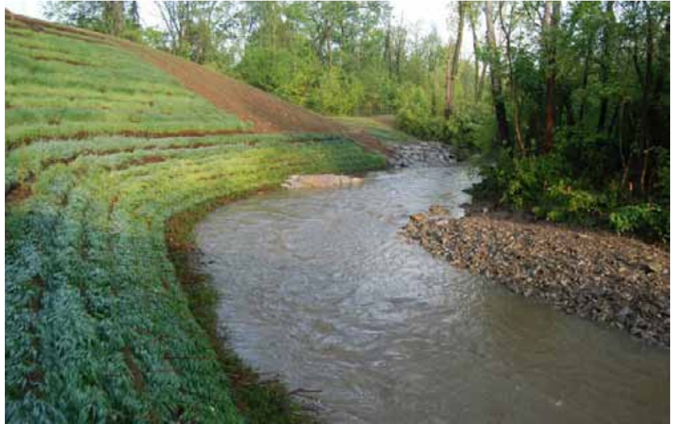
Looking upstream, tall grass provides bank stabilization, June 2012
