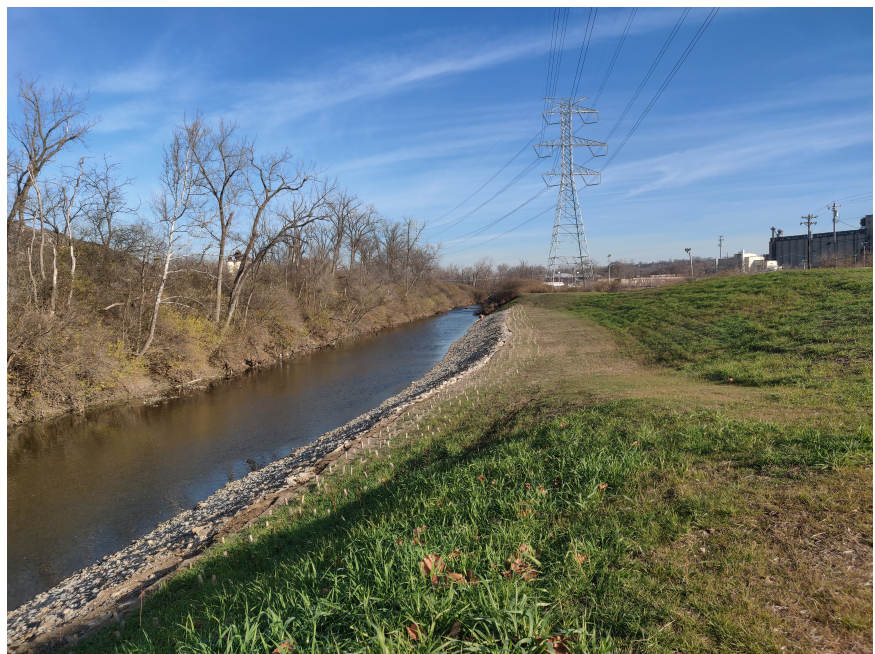
AFTER - Streambank stabilized, open and accessible to public, connected to floodplain, and planted with hardy native floodplain plants
