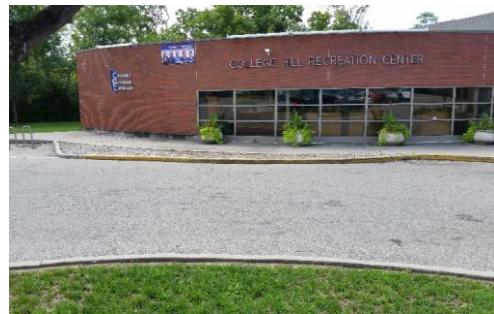
Above: The existing planters at the entrance to the CHRC.
