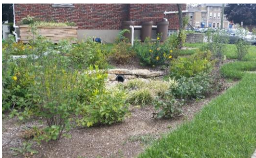
Above: Bioretention facilities are attractive landscape features that provide a critically important function in managing stormwater in urban areas.
